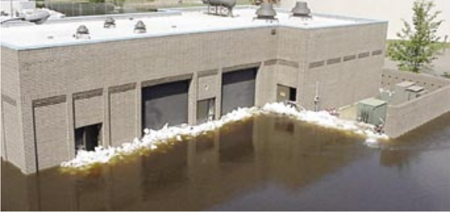
Figure 3. Greenville Utilities water treatment plant surrounded by floodwaters. September, 1999 (Photo courtesy of Greenville Utilities Commission).
