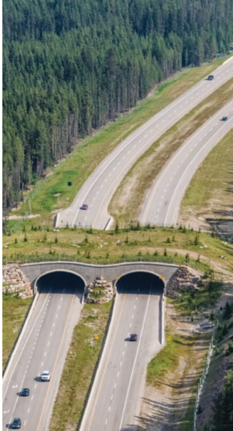
Efforts to improve connectivity in Banff National Park include building overpasses that enable wildlife to safely cross the Trans-Canada highway.
